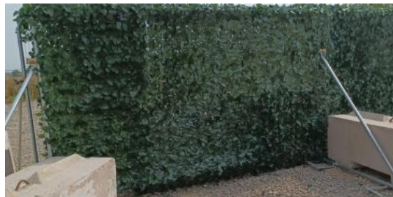
Plate 3.4 Herras fencing with attached textured plastic hedgerow
